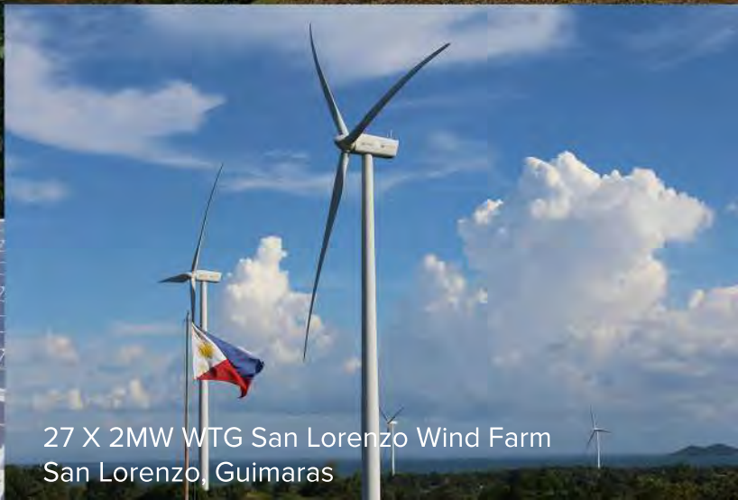
27 X 2MW WTG Pililla Wind Energy Project Pililla, Rizal
